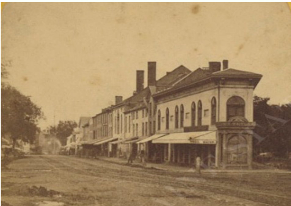
An early view of Congress Street, immediately east of Congress Square. The street is lined with small-scale, two- and three-story commercial buildings.
