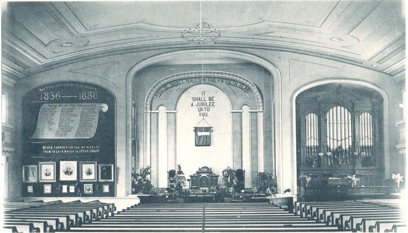
This interior view of the Free Street Baptist Church was published in 1887.
