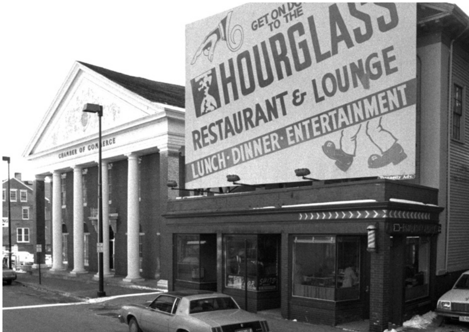
142 Free Street (left) and the former WCTU building at 150 Free Street (right) on January 30, 1980. The WCTU building was torn down later that year.
