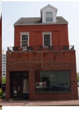
128 Free Street (extant; non-contributing)
